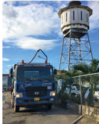
Water tanker truck refilling at WK Plein Water Treatment Plant in Paramaribo; on the right hand side, the old water tower, symbol of SWM.
