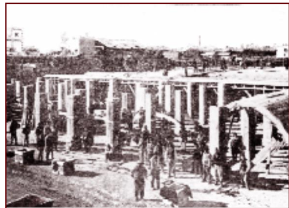
Water tank from Cotroceni under execution (1890)
