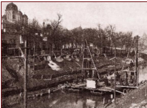
Dâmbovița - sewerage works (1883)
